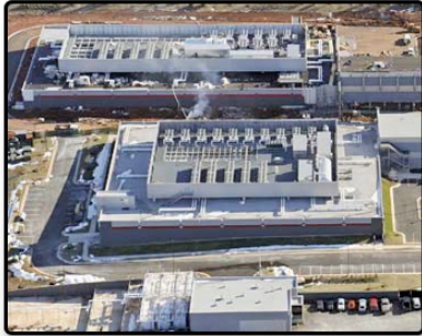
Terremark Data Center
